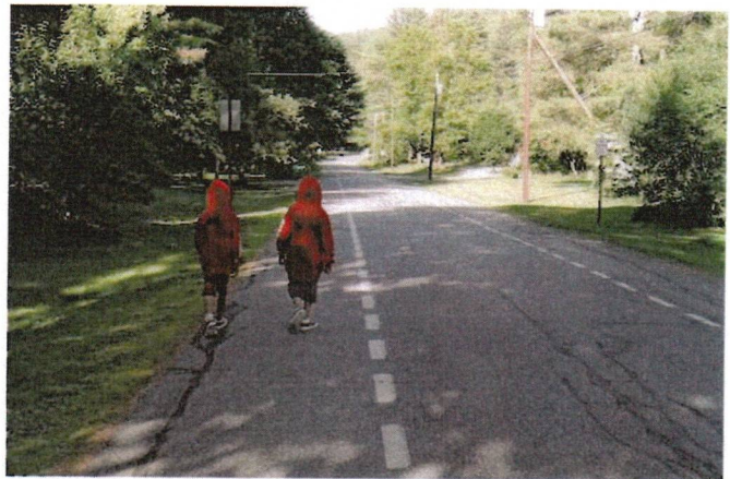
An example of an advisory lane on a narrow road that does not have space for a dedicated pedestrian lane. Photo source: Small Town and Rural Design Guide.
