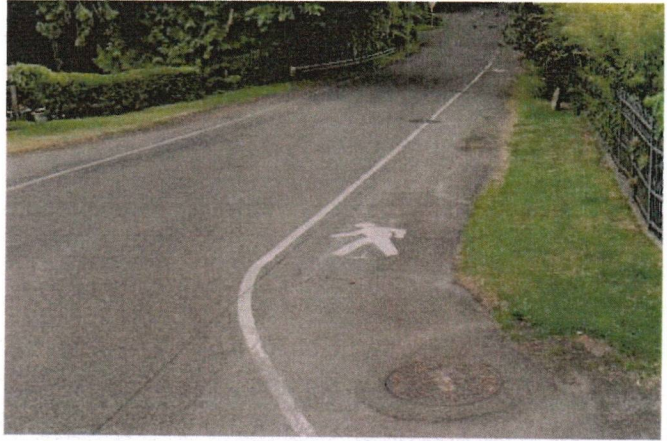
An example of a painted pedestrian lane with a pedestrian symbol in the lane. Photo source: Small Town and Rural Design Guide.
